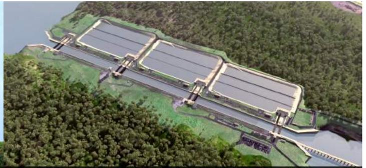
Artist's rendering of Water Saving Basins – the largest in the world. They save and reuse 60 percent of the fresh water needed to operate the lock system. The operating capacity of three basins is 100 million gallons.
