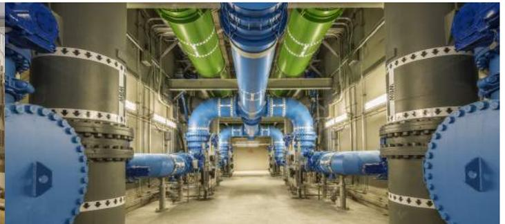
Pipe gallery in the filter building where raw water is filtered as part of the treatment process to produce clean water for the City of Austin. Photo by Joel Crimes.
