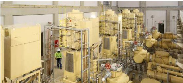
The raw water pump station houses five 375-foot (114 m) lifts, 12.5 MCD, 1,500 Hp vertical turbine pumps. Photo by Travis Bush.
